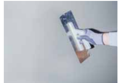
Figure 3 Application of the second layer of the plaster mortar is completed after waiting for slight dehydration of the first layer depending on weather conditions.
