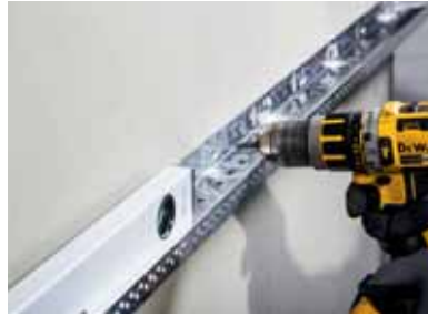
Figure 2 After the leveling process, Teknosistem Socle Profiles are mounted using wall plugs.
