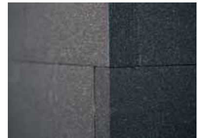
Figure 3 Thermal insulation boards are placed without gaps and in zigzag style upwards starting from the bottom of the wall. Boards should be placed in zigzag style on the corners as well.
