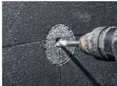
Figure 2 The location of the wall plug is drilled. The size of the hole should be 1 cm larger than the size of wall plug.
