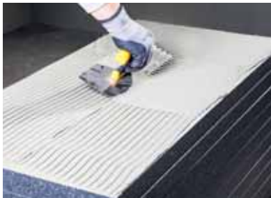
Figure 1 If the surface is flat; the adhesive mortar is applied on the whole thermal insulation board with a trowel or suitably notched trowel, using the method for adhering on the whole surface.
