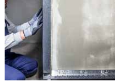
Figure 3 The dimensions of the socle profiles, which should be mounted with a gap of 2-3 mm between them, are selected based on the thickness of the thermal insulation board to be used.
