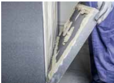
Figure 1 The thermal insulation board with adhesive mortar is applied to its back should be placed onto the socle profile without any gaps.
