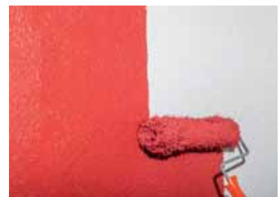
Figure 3 Finally, exterior wall lining and painting is applied.
